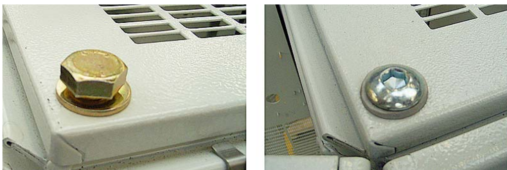
Figure 3-10 Delivery state (left), original roof screws (right)
